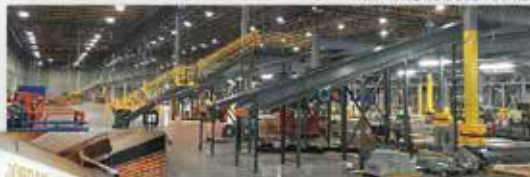
Walmart Distribution Center
